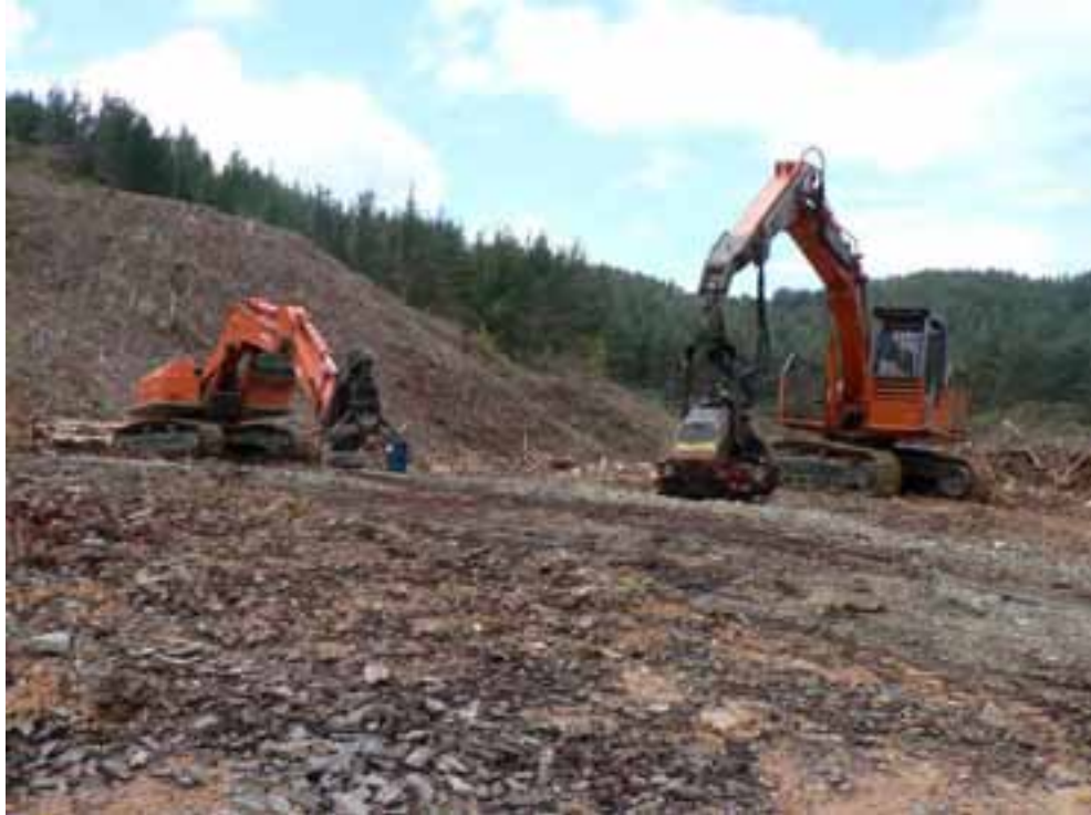
Site EP3: Skidder pad in active logging area in Oweru catchment.
