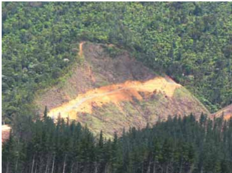
Photo 2: Access roads to extract the logs, are also vulnerable to sediment erosion and may act as conduits for sediment laden runoff directly to streams.
