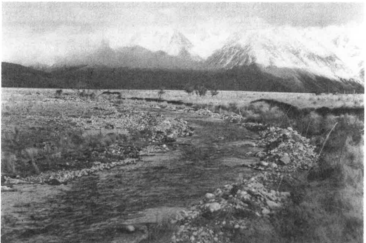
Manuka Point stream improvement. (Note the willow poles at the edge of the new stream.)
