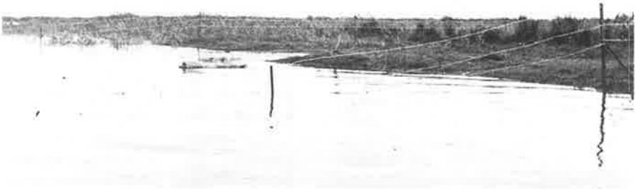
A fence erected on the banks of the Manawatu River in the 1930s to exclude cattle from whitebait spawning grounds.
