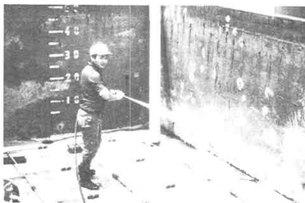
Fig. 9: Cleaning an algal rearing pond. Note the grid of air stones on the bottom of the pond. The figures refer to tonnes of sea water.
