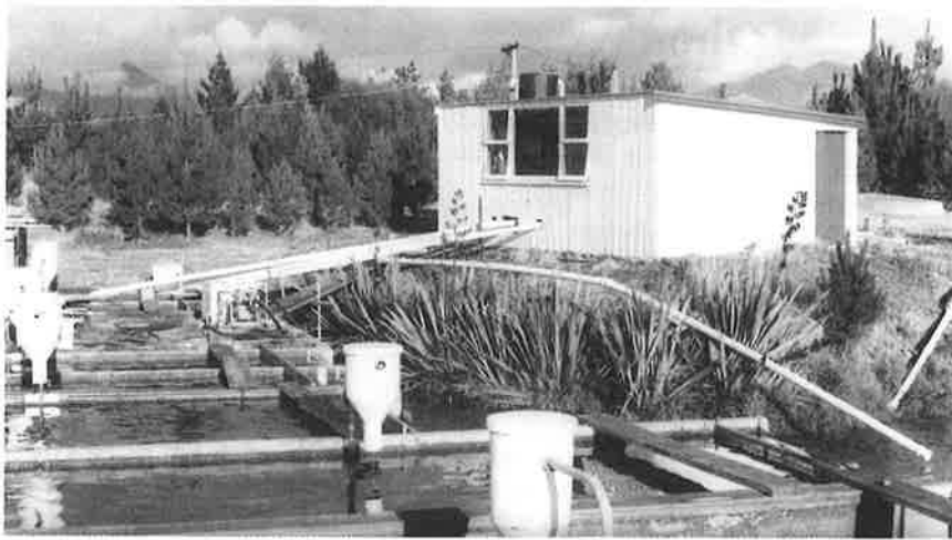
Fig. 3: The tagging shed at Glenariffe hatchery. The pipes leading from the shed to the raceways are connected directly to the tagging machines inside the shed, so that tagged fish are immediately returned to the raceways.
