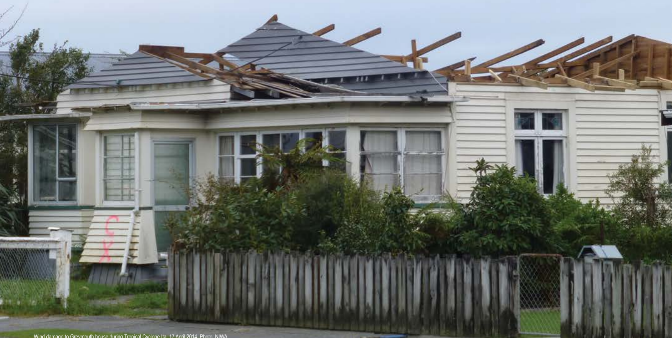
Wind damage to Greymouth house during Tropical Cyclone Ita, 17 April 2014. Photo: NIWA.
