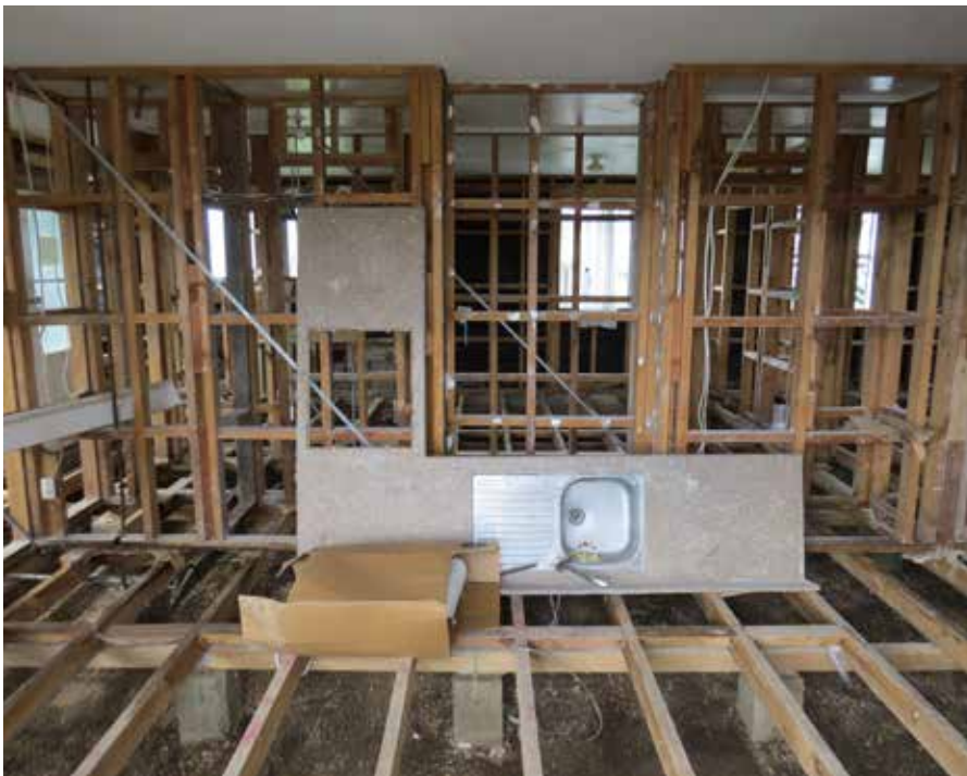
Interior house damage. Source: NIWA
