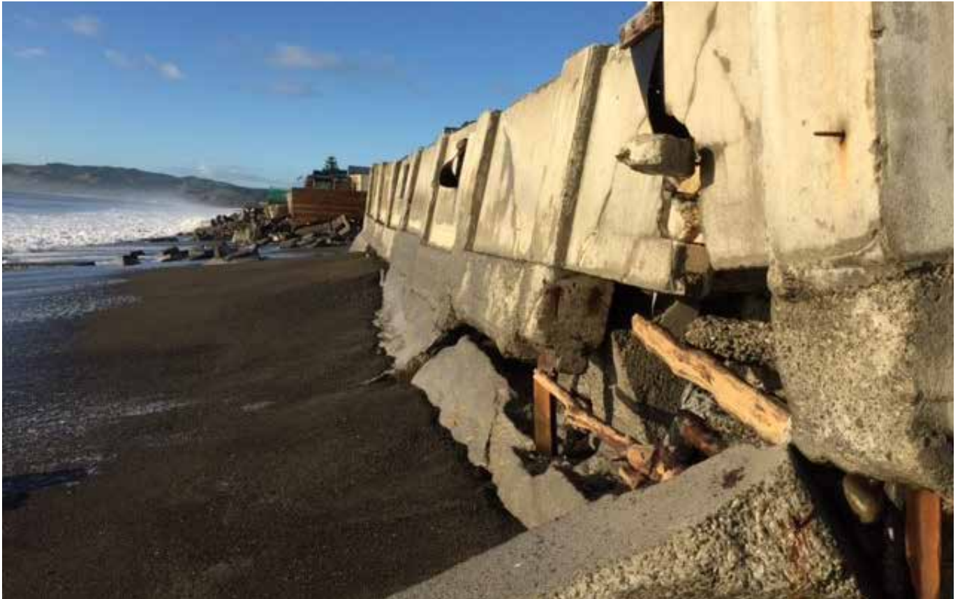
Broken and undermined seawall at Haumoana, Hawke's Bay after a large swell event in July 2017.
