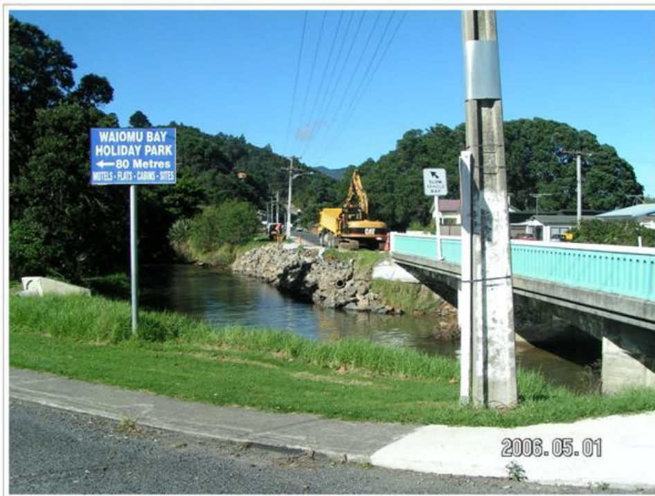
4 Recent erosion protection works placed by Transit
