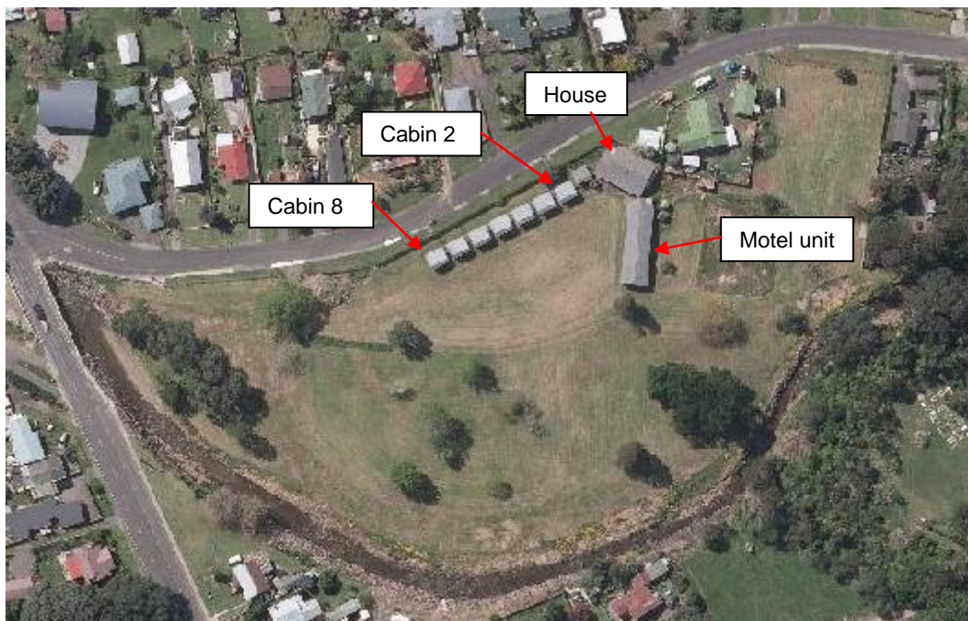
Figure 23 Existing buildings retained on site
