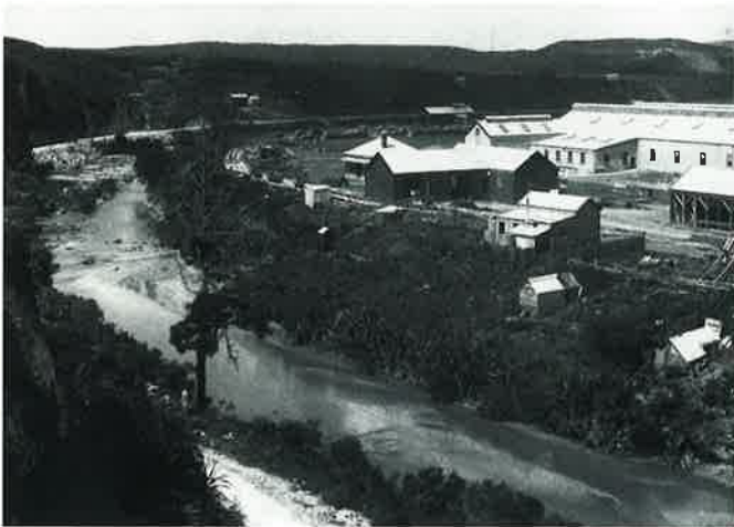
Gold ore processing plant next to the Ohinemuri River in the early 1900s. (Photo: Alexander Turnbull Library)
