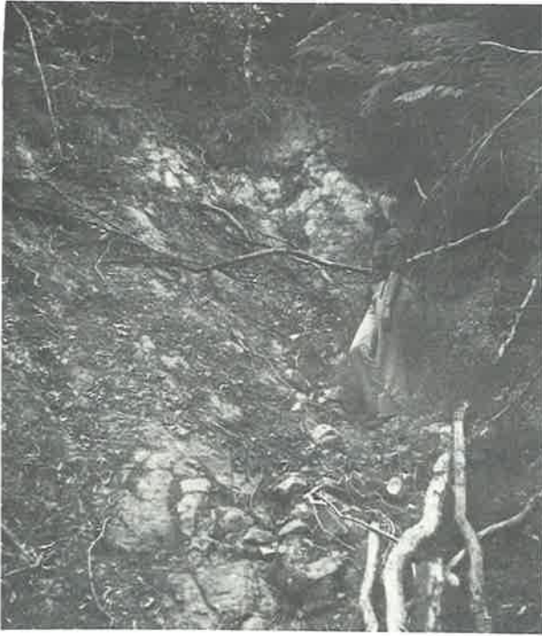
Photo 1 —Natural slip in gully head situation with shear plane along contact between bedrock and regolith.
