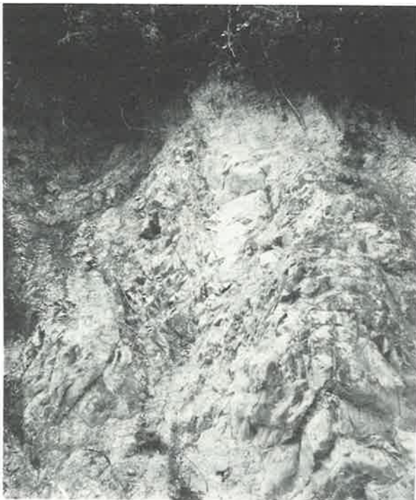
Photo 3 —Bedrock failure among joint planes in a cut slope—note range of jointing.
