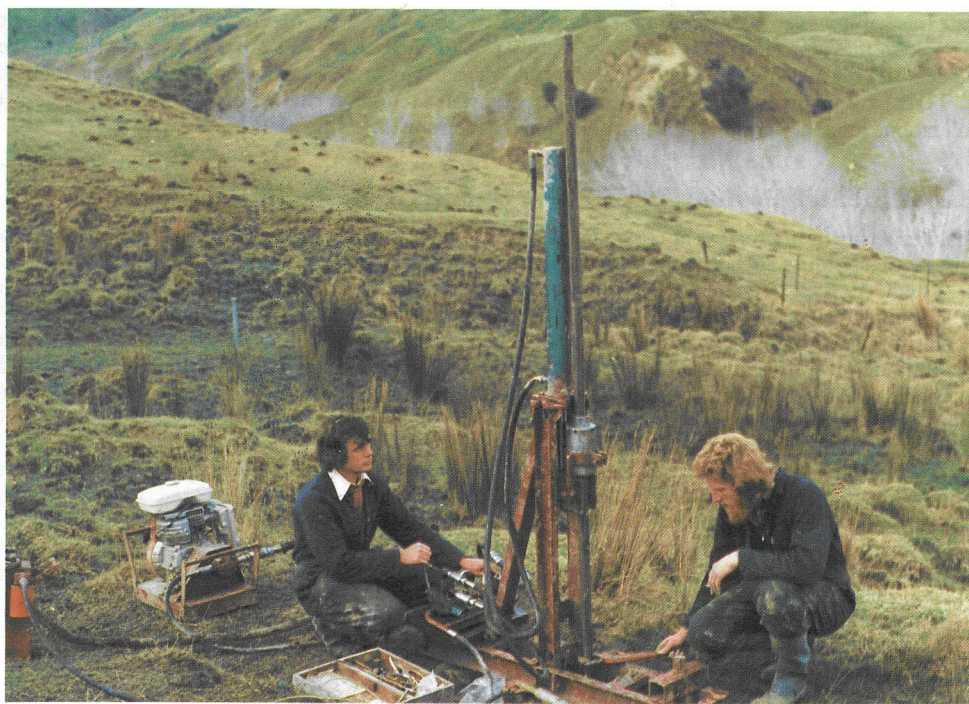
Fig. 12 Deep soil sampling using motorised equipment designed by the Land Stability Group.
