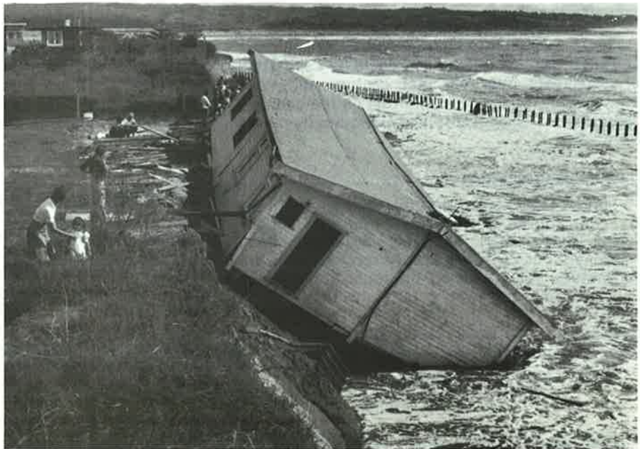
FIGURE 5. Ohiwa Spit looking west towards the entrance with Ohope in the background. Attack by heavy seas on 18–21 April 1976 caused severe erosion resulting in this house collapsing into the sea. Note the line of rails in the sea. These were placed along the dune toe in 1970 as coastal protection. Photo taken 21 April 1976 by R.K. Smith.
