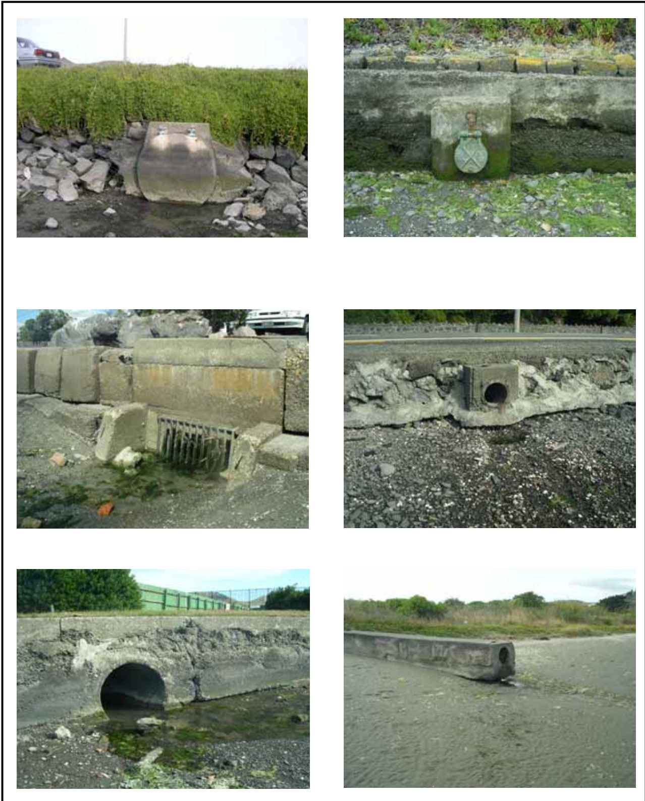
Figure 2.3 A representative sample of the outlets through which stormwater is discharged directly into the Avon-Heathcote Estuary/Ihutai
