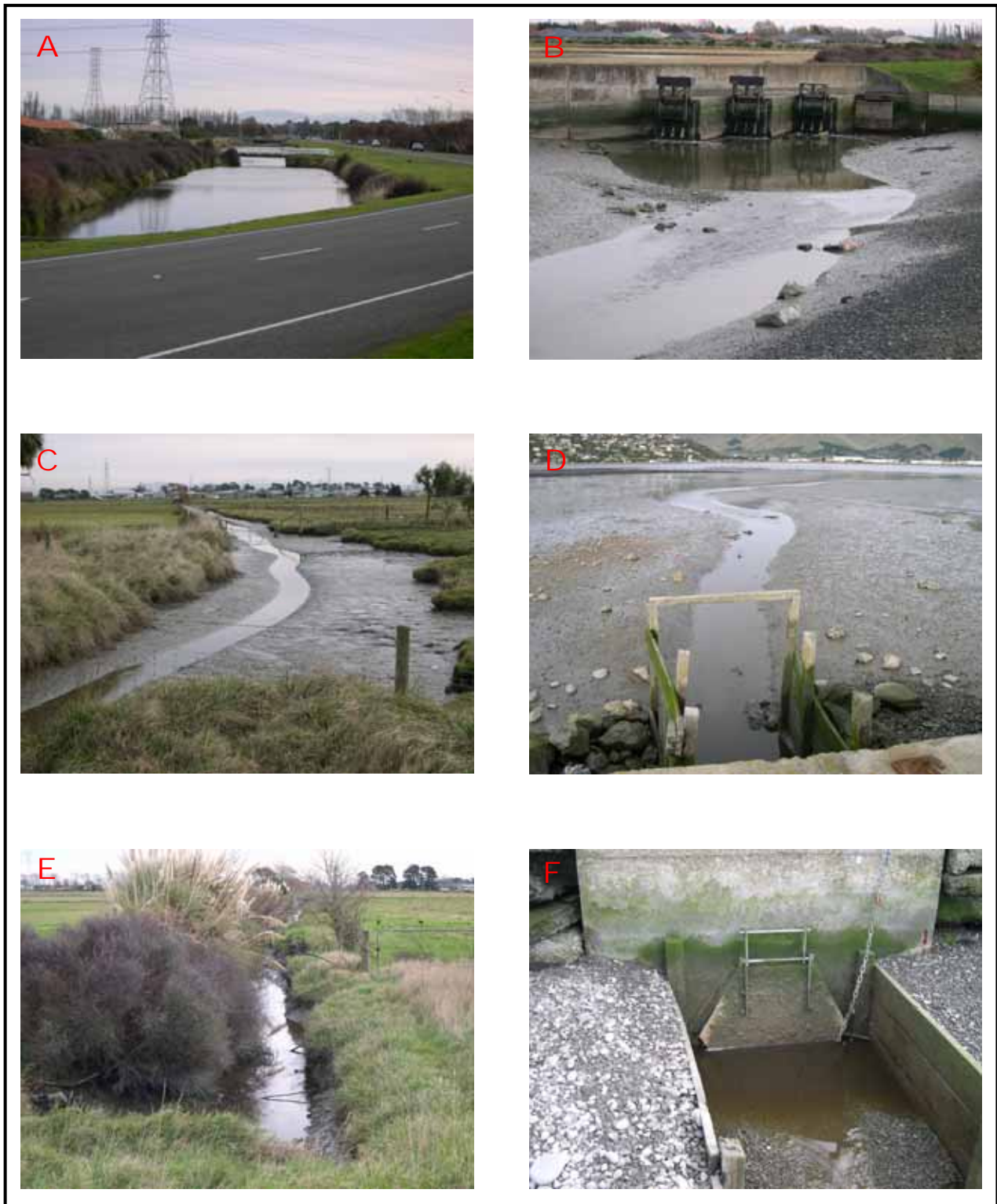
Figure 2.2 Three of the drains and their outlets into the Avon-Heathcote Estuary/Ihutai
