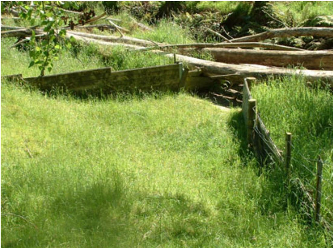
**Photo 4: Gully control flume structure – maintenance required to remove fallen trees**
