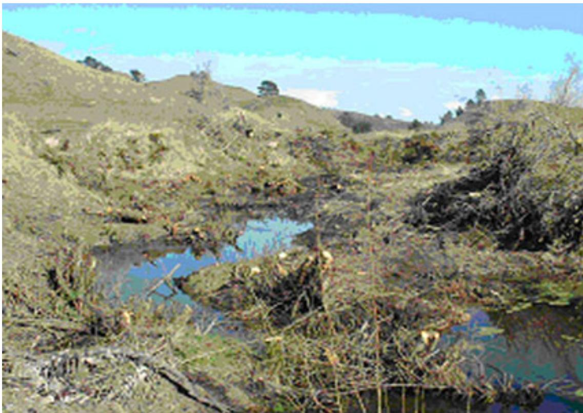
**Photo 6: Stream channel following transitional works to address willow congestion**
