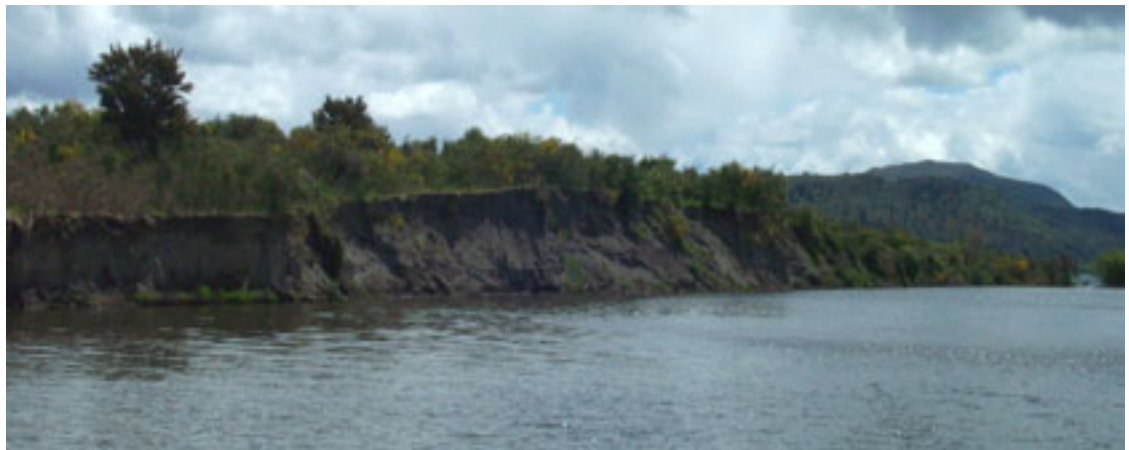
Figure 20: An indication of the volume of floodwaters exiting via Deep Stream is shown by the erosion caused to its left bank before it enters Lake Taupo (near the mouth of the Tokaanu tailrace).
