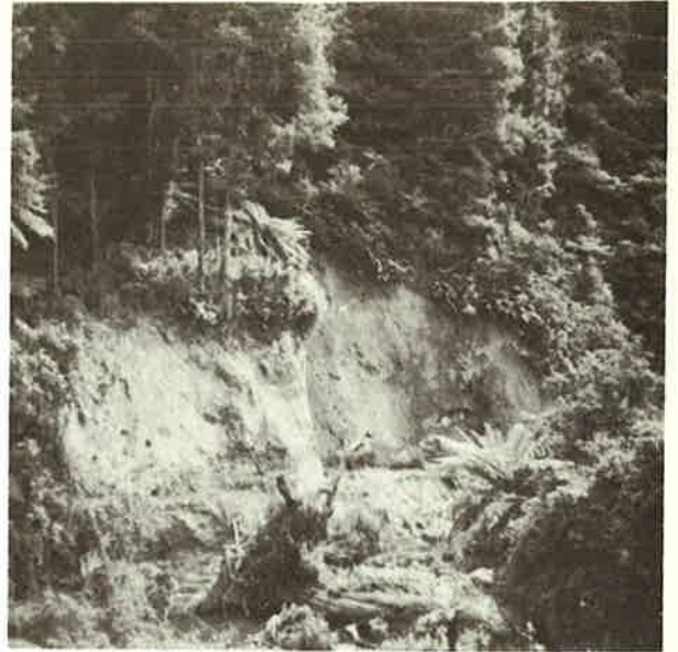
PLATE 6 —Severe bank erosion.
