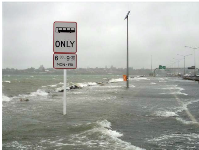
Figure 11. Southbound lanes on Auckland's northern motorway are submerged during a storm that coincided with high tide in January 2011. Source: NZTA
