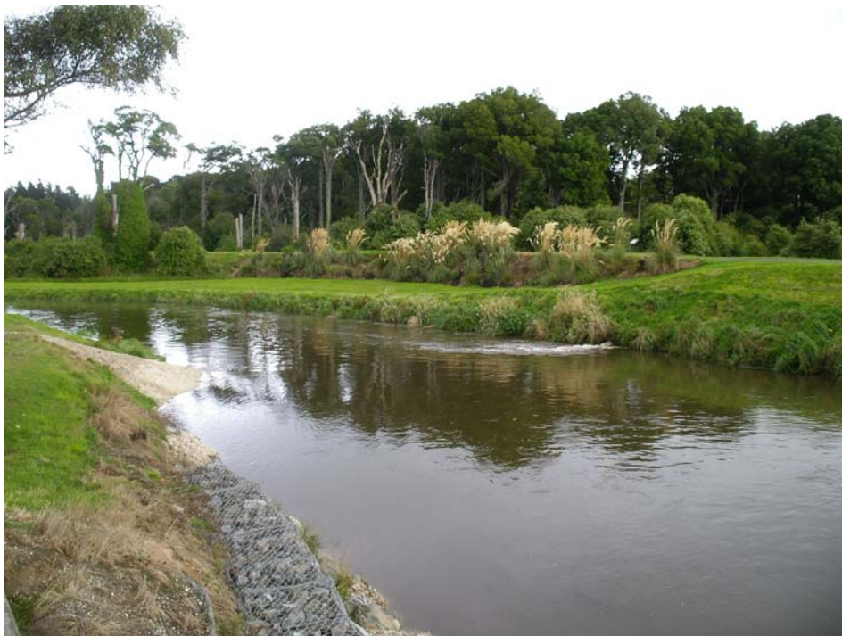
Figure 2.1: Waihopai River, downstream of Queen's Drive Bridge
