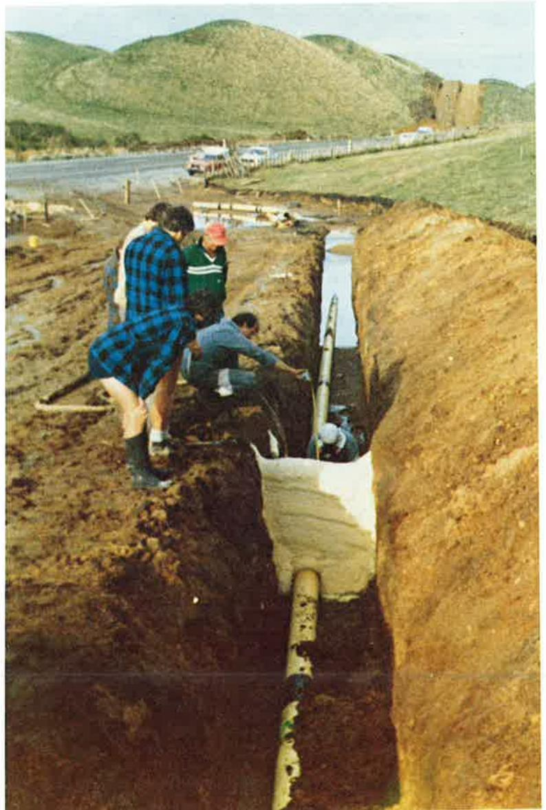
**Figure 5:** Kinleith—Kawerau natural gas line, 1982. Foam breakers can be used to stop water flowing down the trench and to support backfill material.
