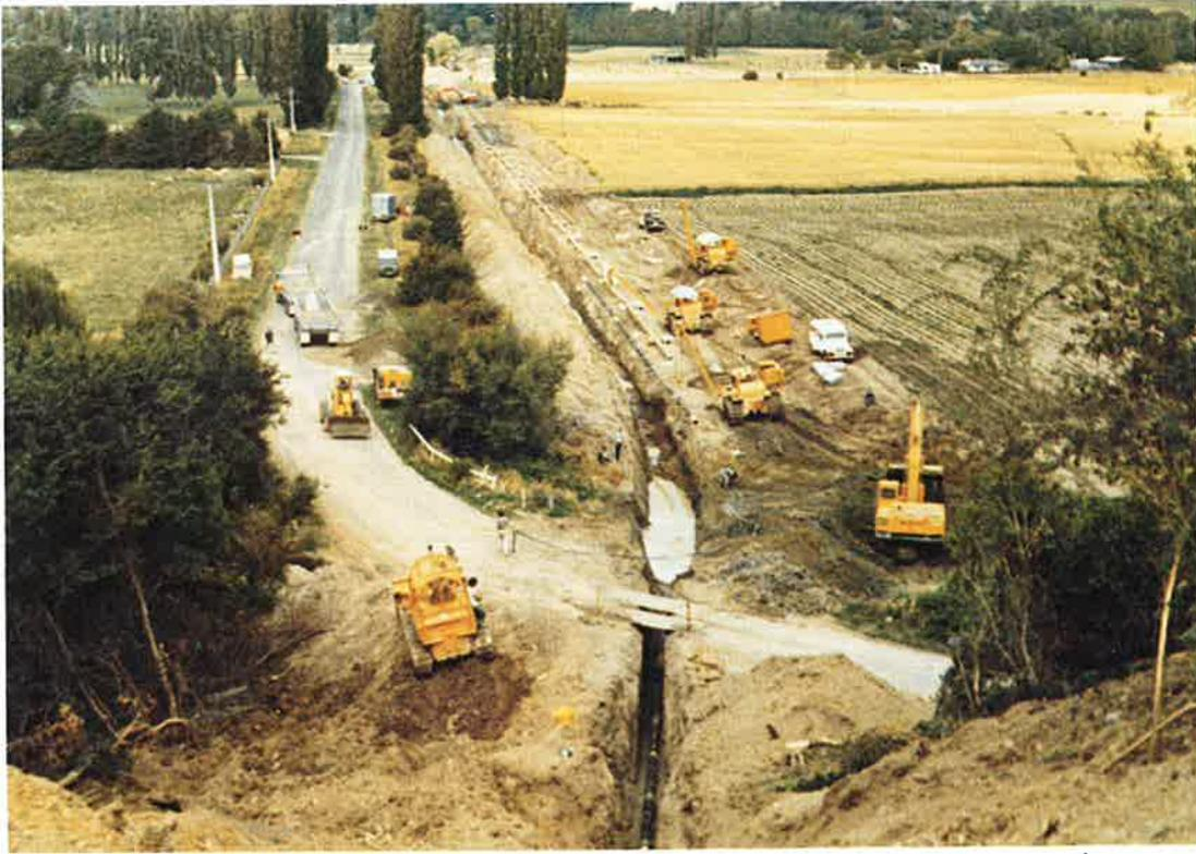
**Figure 4:** A section of the Hawkes Bay natural gas line being laid near Ashhurst, 1983. Note the problems of using a restricted right-of-way through areas of cropping. Vehicles damage the topsoil by using it to gain access to the line.
