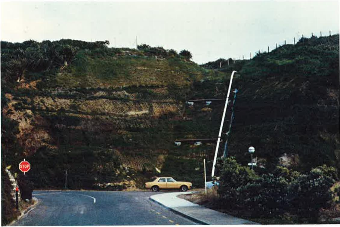
**Figure 8:** Port loading line, New Plymouth, 1983. This face was difficult to reinstate. The top section, which is sand, was covered with plastic mesh and a wood fibre mulch and then seeded. The lower section was hydroseeded. The bench drains were planted with flax.
