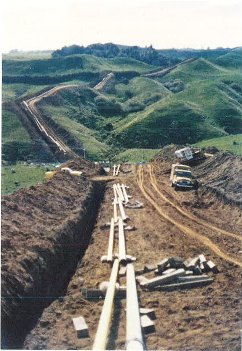
**Figure 2:** McKee oil lines near New Plymouth, 1984. Note the stockpile of topsoil on one side and trenching material of subsoil on the other, with the trench and the right-of-way between. Access to the right-of-way is had by leaving a gap in the stockpile of subsoil and a plug in the trench.
